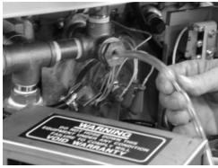
Feed the tubing through the access port in the boiler compartment.
